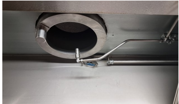
Opening with collar fitted and grease-collection nozzle connected at the lower edge.
