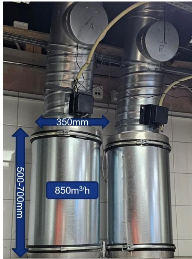
Two Lynx Kitchen units mounted above a kitchen hood. Dimensions: 350 mm diameter, 500–700 mm height, 850 m 3 /h per unit
