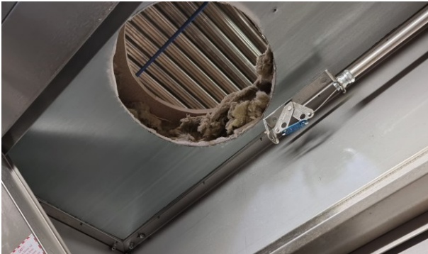
A 360 mm opening cut into the hood top plate.
