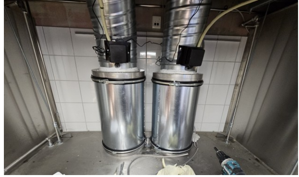
Two Lynx units with converter boxes mounted, clamp ring ready for fitting.
