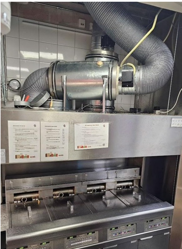
Horizontal Lynx Kitchen installation.
